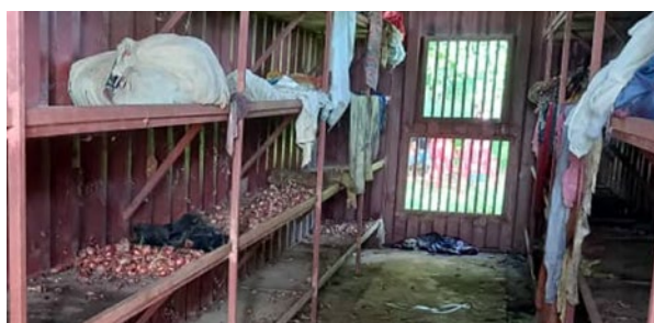
40-foot Freight Container Converted into an Onion Curing Facility, Foni Brefet, The Gambia
