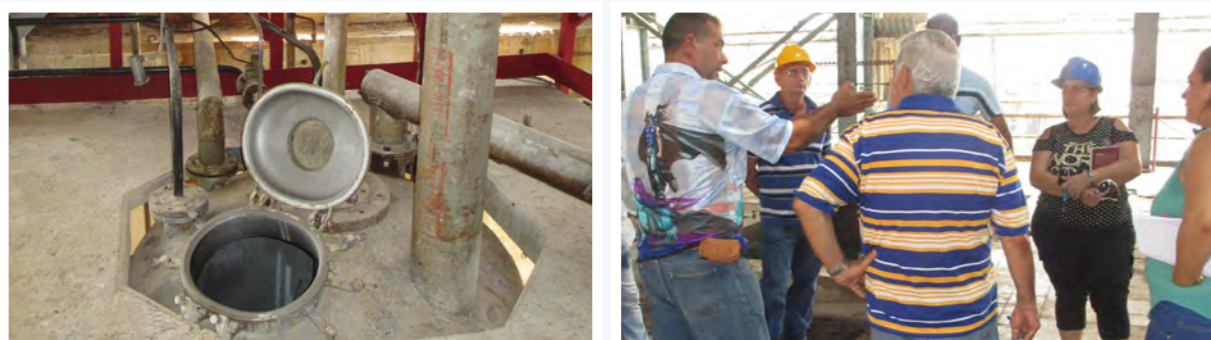
Figure 14: Refurbishment process at the calcium nitrate production plant in EMPREQUIN, Nuevitas
